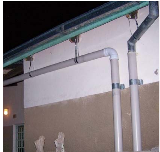
Rain gutters were added to the orphanage.
